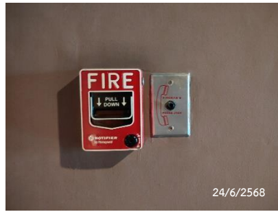
Fire Alarm Manual Station
