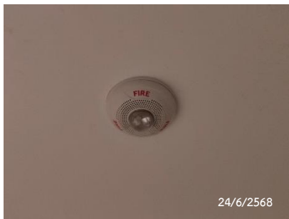
Fire Alarm Horn Strobe
